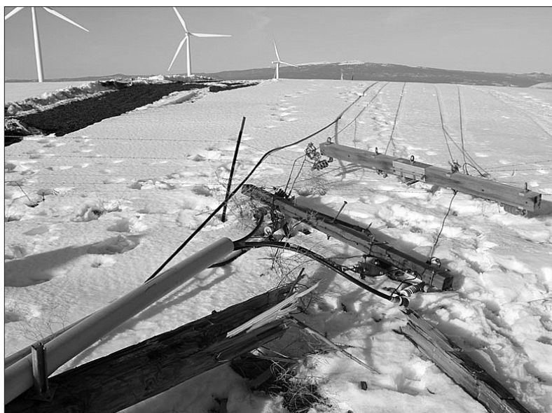
Snow and freezing rain together make a treacherous combination to power lines and poles. Four other utilities came to KPUD's aid during this large storm in 2012.
