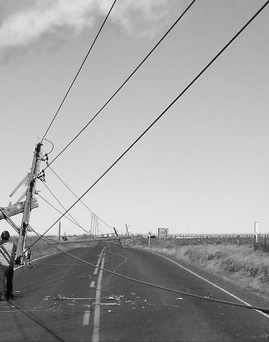
Inhospitable weather in Klickitat County comes in many forms. Multiple poles came down in a windstorm in the eastern part of the county. All KPUD crews responded and restored power in record time.
